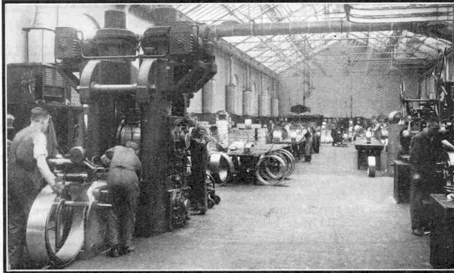
Fig. 3. Rolling stainless steel strip for aircraft manufacture.
