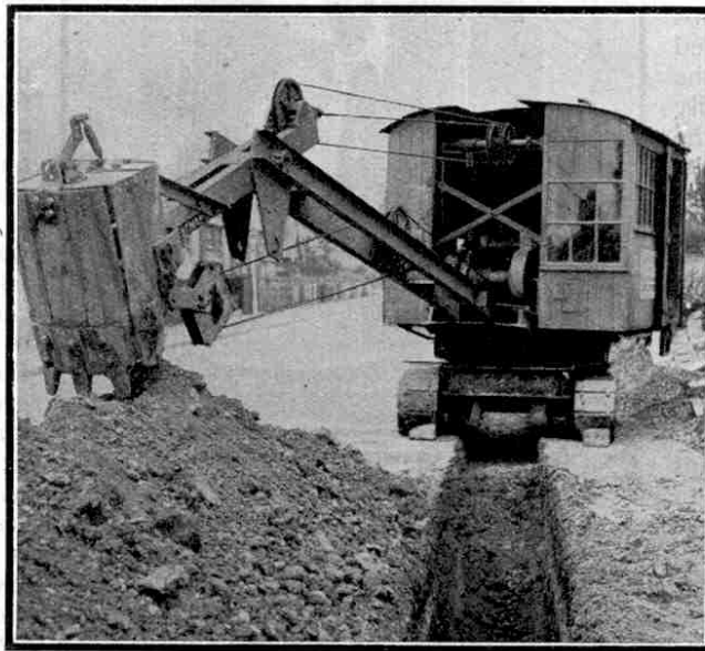
Cutting a trench through hard gravel with the aid of a "Universal" Trench Shovel.
