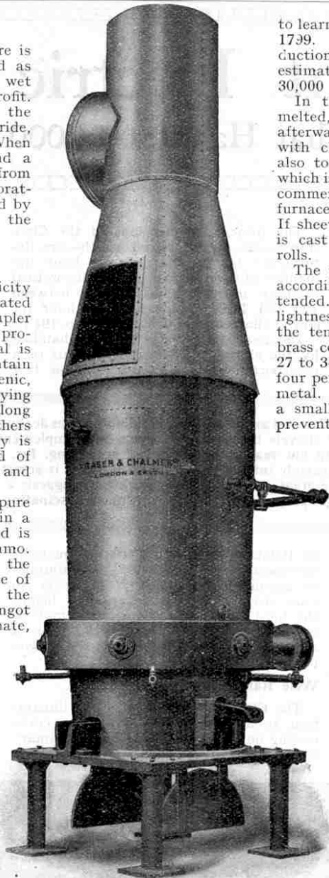
Copper Blast Furnace, circular type
