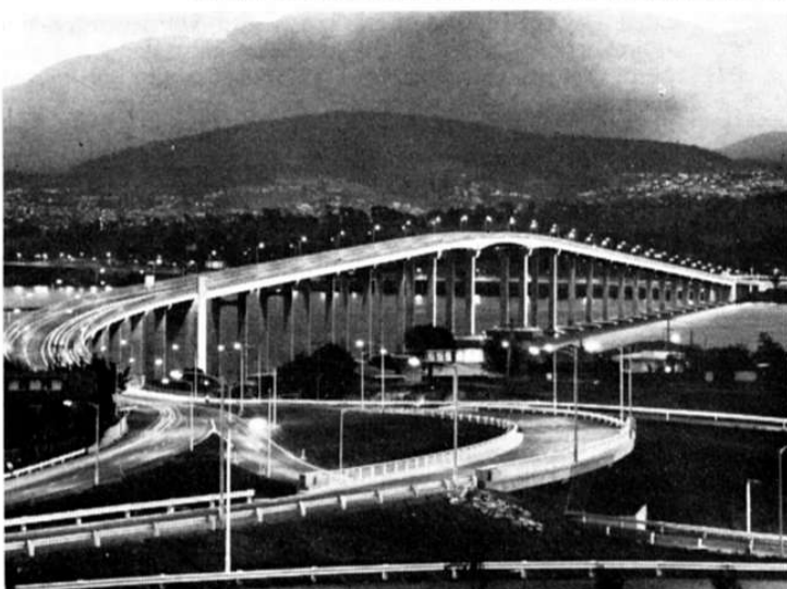
Below, left, the Tasman Bridge crossing the Derwent River in Hobart, Tasmania. One of the world's longest prestressed concrete bridges, it was completed in 1964 with a length of about 1100 feet. ( Aust. Info Service ). Below, right, the Batman Bridge, Tasmania, spanning a 225 yard stretch of the Tamar River with a cable cantilever. ( Aust. Info. Service. )
