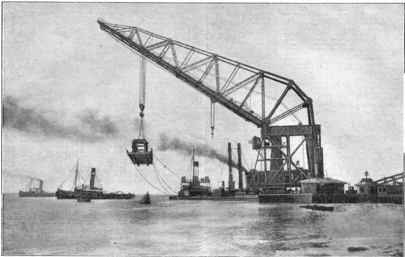
THE 200-TON FLOATING CRANE "MAMMOTH," LIFTING A BRIDGE WEIGHING 152 TONS, AT NEW BRIGHTON FERRY.
