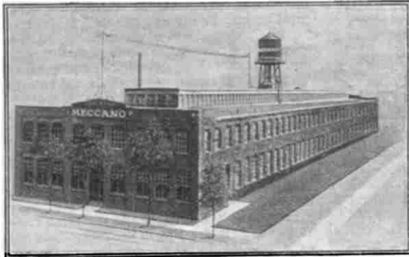
THE NEW MECCANO BUILDING AT ELIZABETH, NEW JERSEY.
