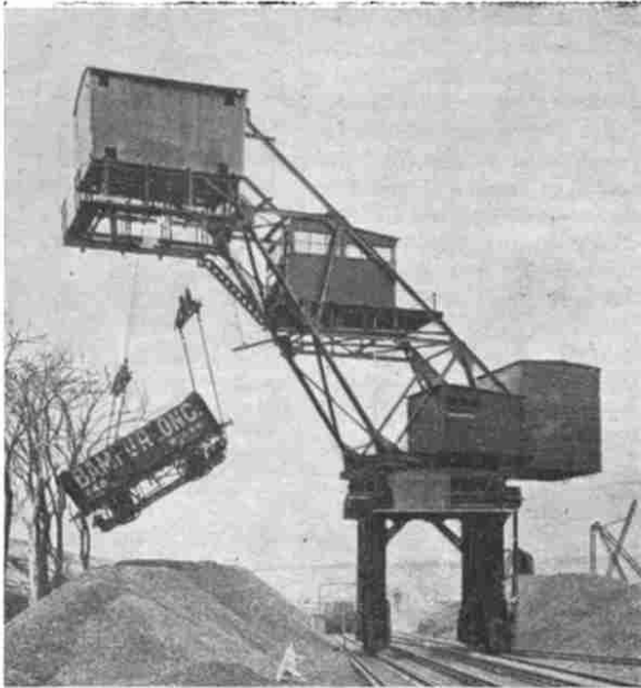
THE MITCHELL APPLIANCE AT BLACKBURN POWER STATION EMPTYING A WAGON.
