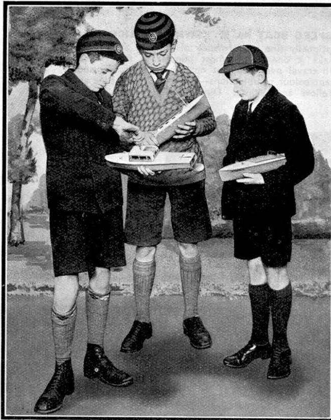
A proud owner demonstrates to his chums the winding of the motor of his Hornby Limousine Speed Boat. The key passes through the roof of the cabin to the winding spindle inside.
