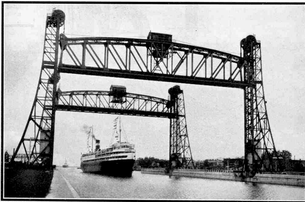
Two of the lift bridges of the Welland Ship Canal open to allow the passage of a large lake steamer entering the Canal from Lake Erie. There are 20 bridges across the Canal, and 10 of them are similar in type to those shown in our photograph. We are indebted to the courtesy of the Department of Railways and Canals, Canada, for the illustrations to this article.
