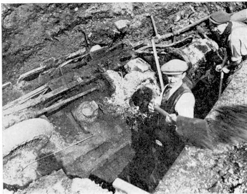
Resurrecting the decayed remains of the Wolseley Gyrocar in 1938.
